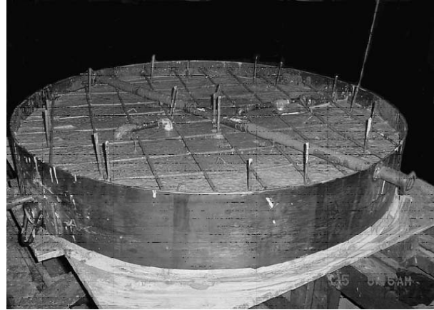
Figure 2. Reinforcement roddings placed inside the metal box
