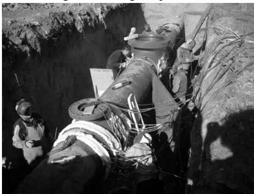
Figure 2. Welding conducting- place Beska
