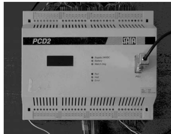
Figure 3. PLC SAIA PCD2
