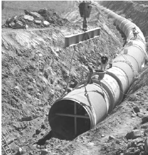
Figure 1. Installation of underground mortar coated steel penstock (by Welded Steel Pipe)
