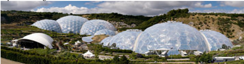
Figure 3. Greenhouse Eden / Nicolas Grimshaw, the use of ETFE-pillows [3]
