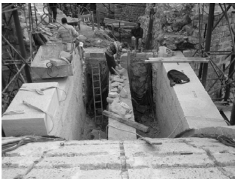
Figure 7. Assembling of the spandrel walls and middle rib
