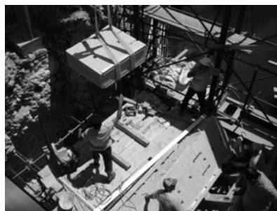
Figure 3. Assembling of the load bearing arch
