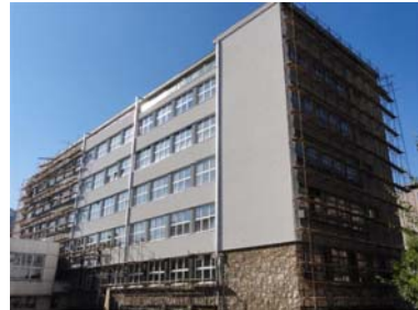
Figure 3. View on the west MEF building after
