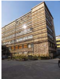
Figure 2. View on the west MEF building before
