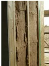
Figure 1. Wood fibre wall insulation in section
